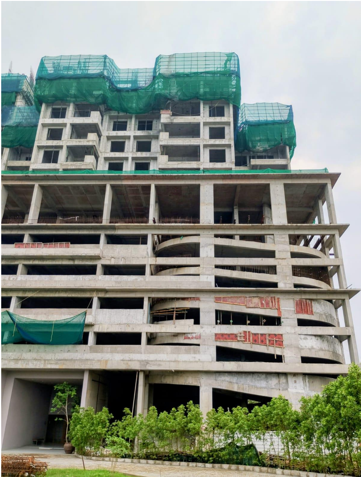
Tower 12 – Super-structure work in progress i.e. 12 th slab work in progress.
